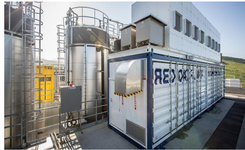
Vanadium Redox Flow Battery
