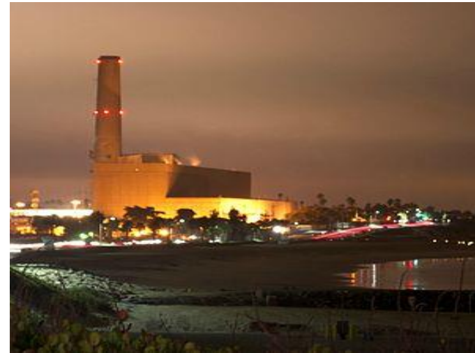
Encina Power Plant
